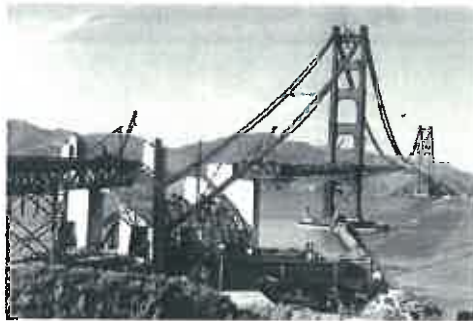
Construction of Golden Gate Bridge
