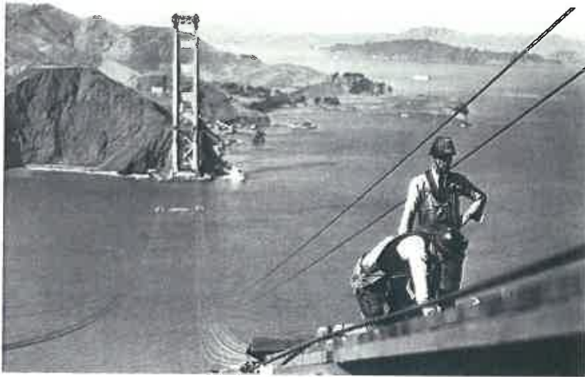
Building Golden Gate Bridge
